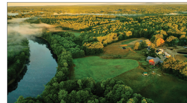
The Ecology School (TES) recently constructed a new campus at River Bend Farm on the banks of the Saco River. The 105-acre campus includes 3.5 miles of walking trails, a 144-bed dormitory, an agroecology farm, and a dining commons. Spectrum began a partnership with TES in 2021.
